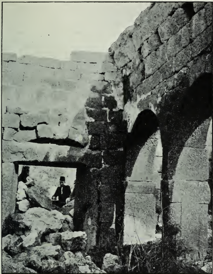
FIG. 223.—Maden Dagh, nave, looking W.
